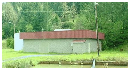
Hayhurst Rd. Treatment Plant
